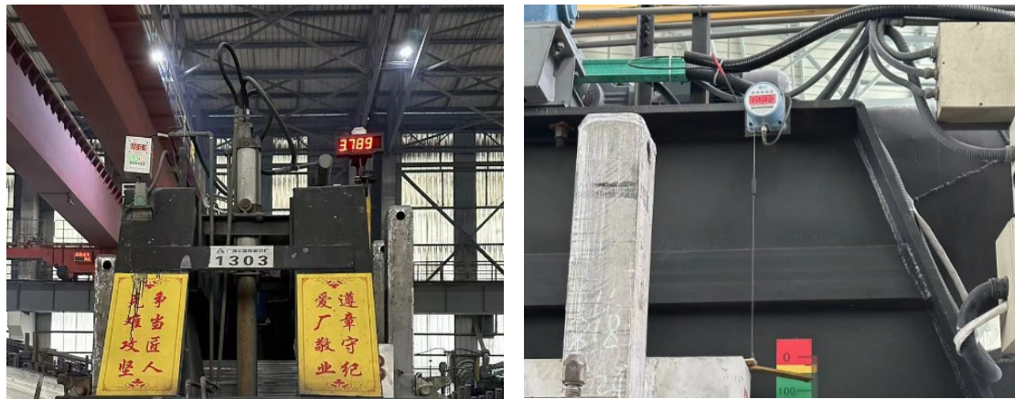
Figure 9. On site installation and application of equipment.
